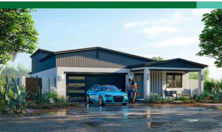
Concrete printed home by Virginia Tech. Chico State NSPDC is proposing acquisition of similar 3D printer.
